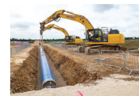
Example image of pipeline installation
