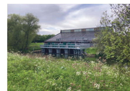
Example image of typical pumping station
