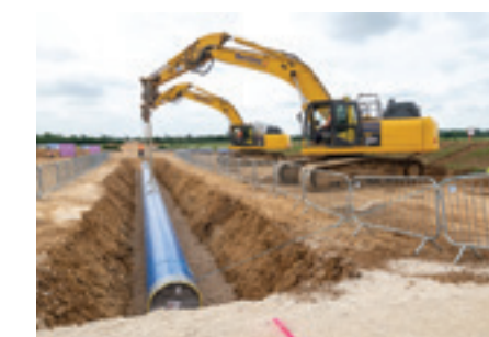
Example image of pipeline installation
