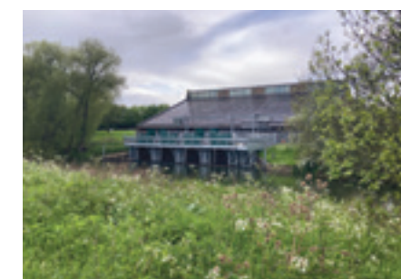
Example image of typical pumping station
