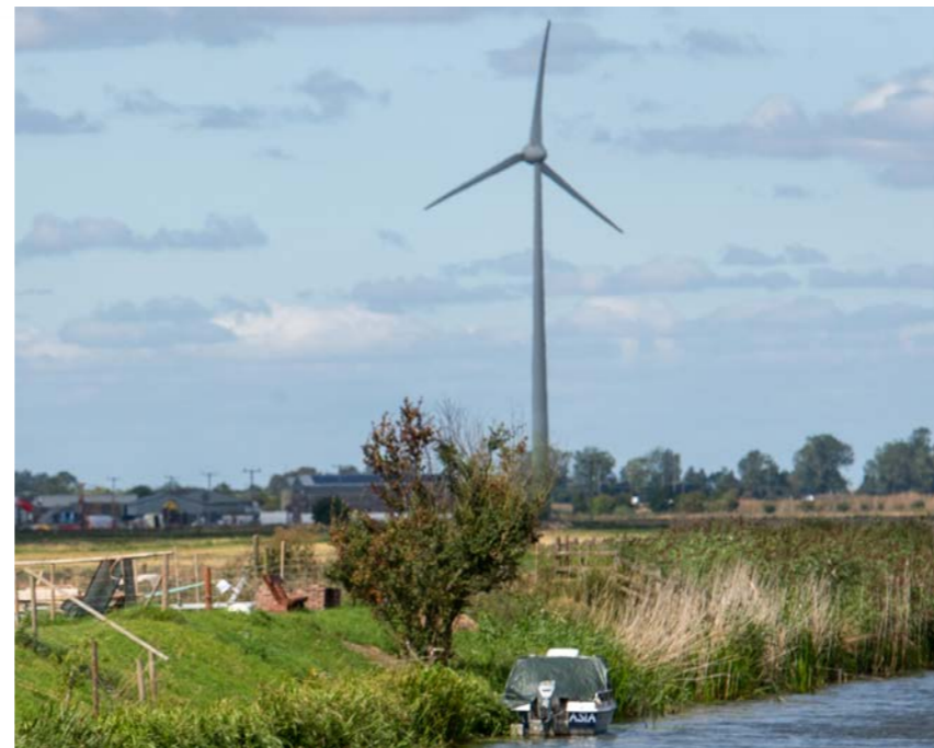
Existing wind turbine to the north of Long Nightlayer’s Drove
