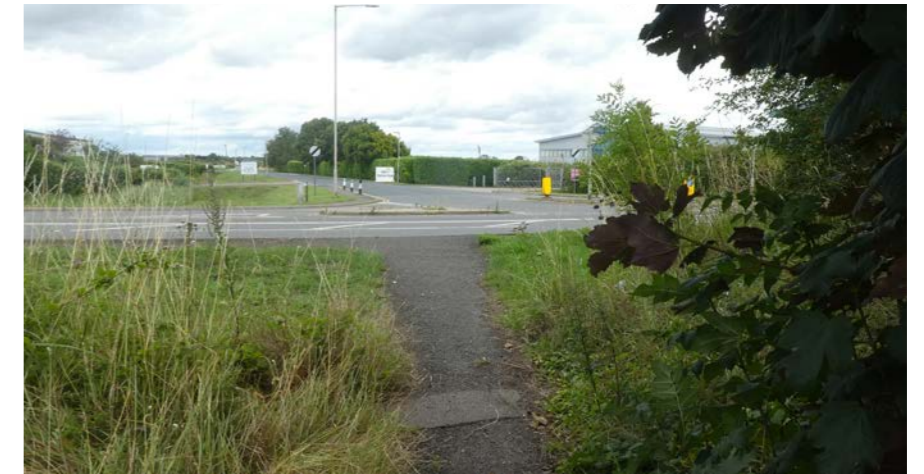
Poor quality crossing point from PRoW south of the A142 to Fenton Way
