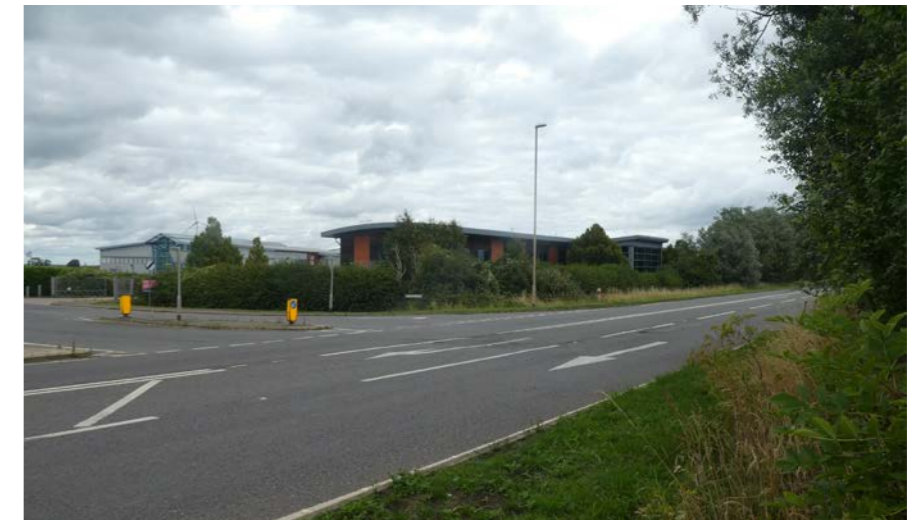
Light industrial development on low land at the northern edge of Chatteris
