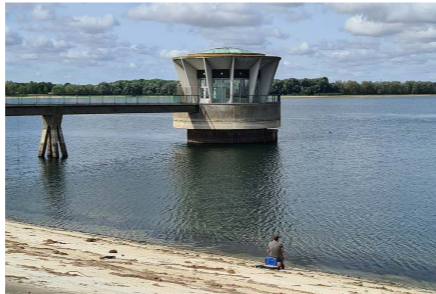
Example of a typical outlet tower and bridge
