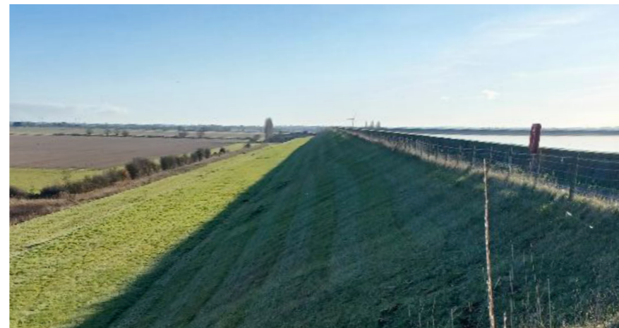
Covenham Reservoir - An example of a standard non-impounding reservoir. This approach would not meet the requirements of the NPS which will apply to the Fens Reservoir
