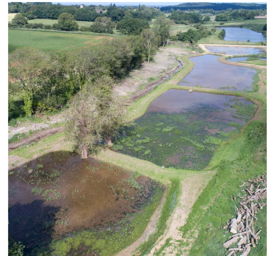
Example of wetland creation to improve water quality in the River Ingol at Ingoldisthorpe
