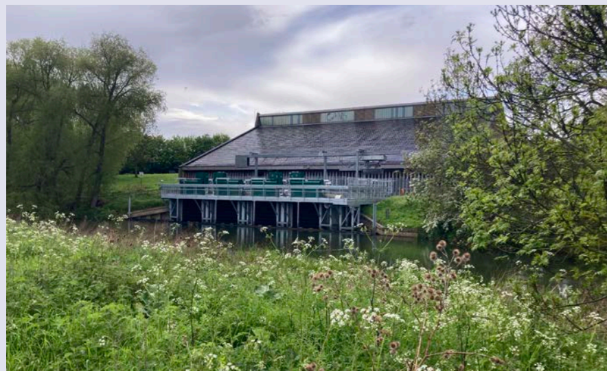
Example of a pumping station at Tinwell
