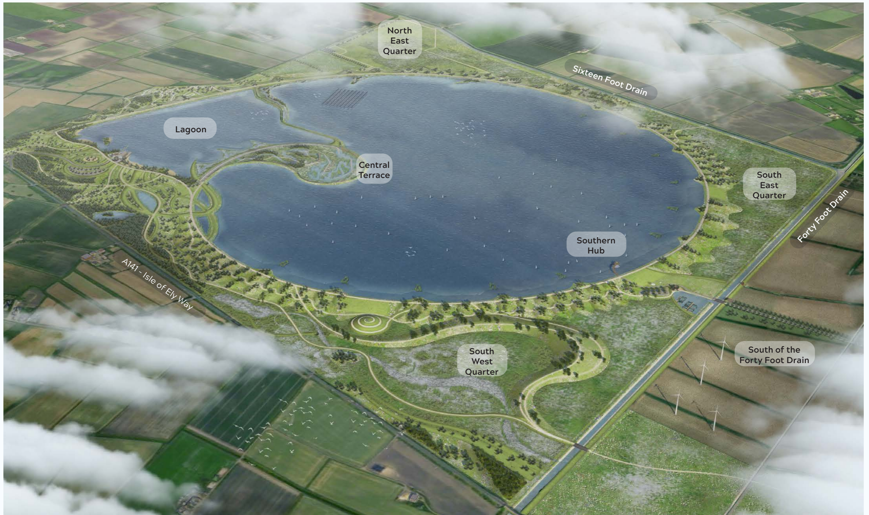
Approximate locations of component areas indicated on artist's impression of the reservoir from the south-west
